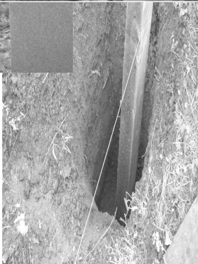
badger and the stamina of a thoroughbred, each post hole is dug by hand to a spade's length depth. Each rail measured and set straight – every angle and gradient checked and assessed. Keep it up chaps, we might see if finished before the end of the magazine... The PCC thank John Hembrow for allowing access and use of his field whilst work was undertaken.
